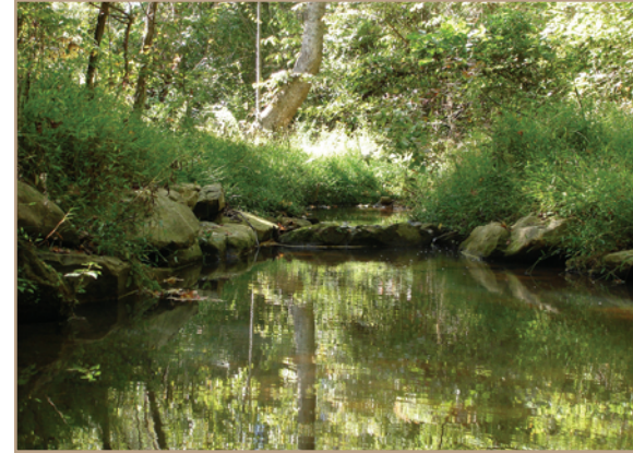
▲ Constructed riffle with rock vane to dissipate flow energy, provide grade control, and enhance aquatic habitat.
